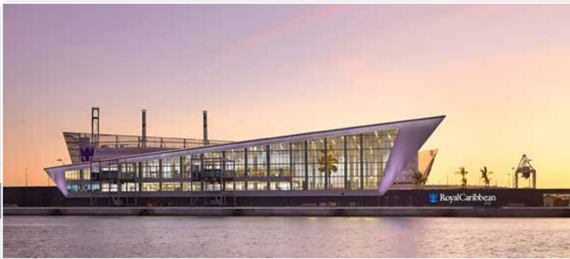
Royal Caribbean Terminal A at PortMiami, which CTI owns and operates, opened in 2024.
